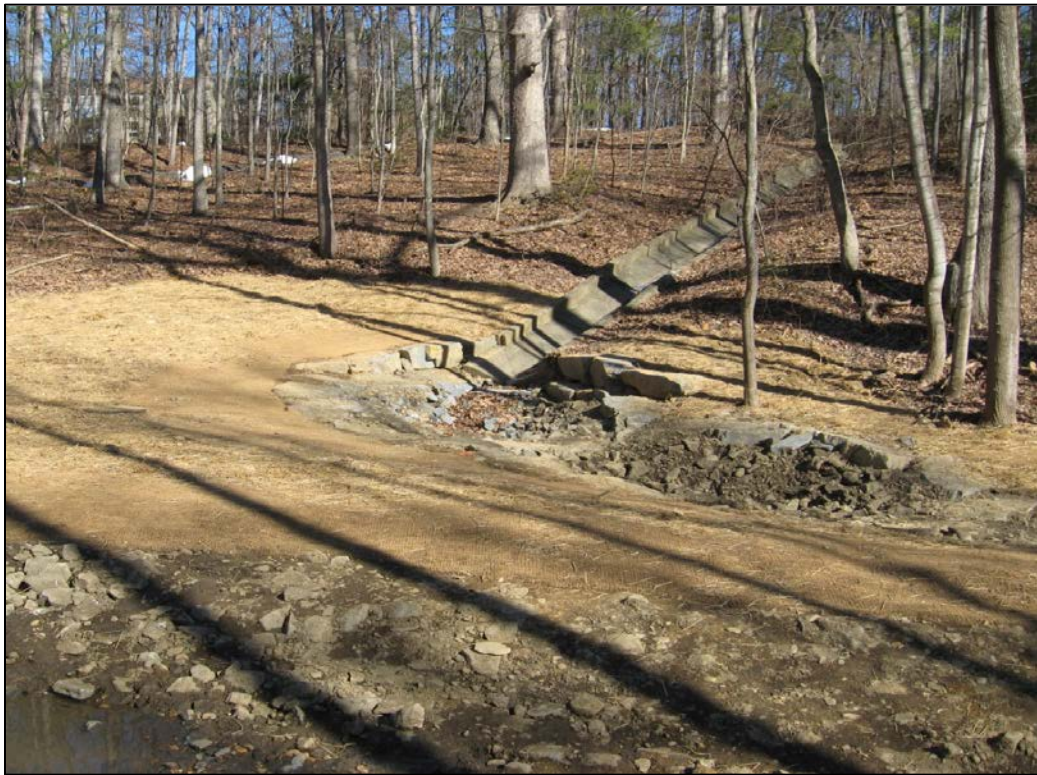
Confluence has been shifted away from the manhole that was exposed prior to restoration.
