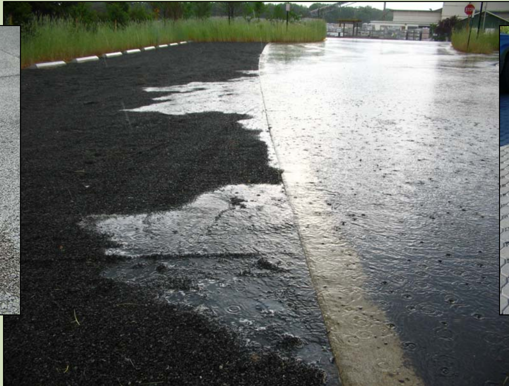
GravelPave2 infiltrating a large rainstorm at WSSI
