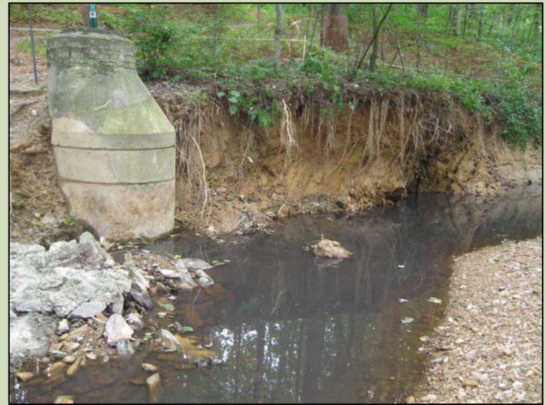
Exposed sewer manhole – Reach 12 in Snakeden
