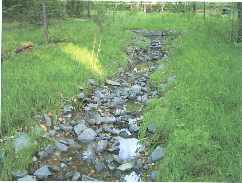
Photo 1 – Looking upstream at affected riffle prior to repair. Small head-cut is visible toward the top of the riffle.
