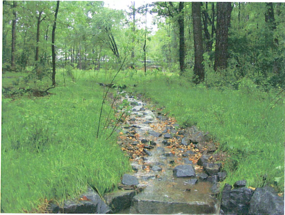
Photo 3 – Looking upstream at affected riffle after repair and additional rain event of approximately 0.75". Bed remained stable.
