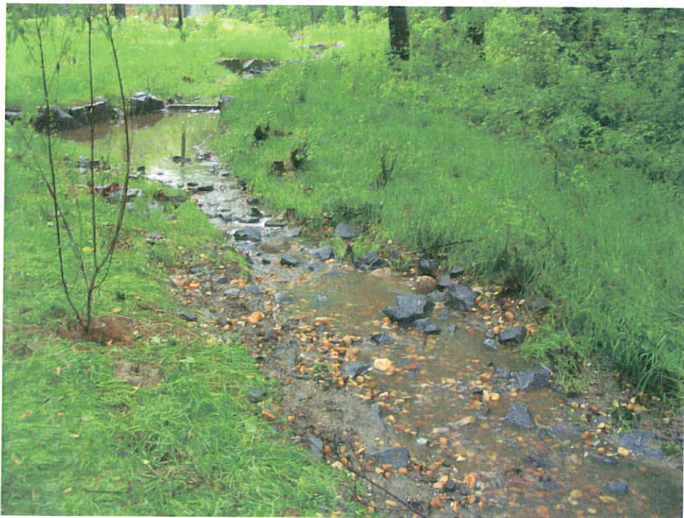
Photo 4 – Looking upstream at previous head-cut after repair and additional rain event of approximately 0.75". Bed remained stable.
