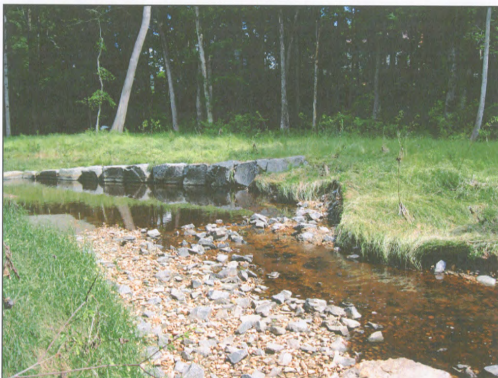
Photo 2 – Erosion along left bank below structure, likely due to improper grading.
