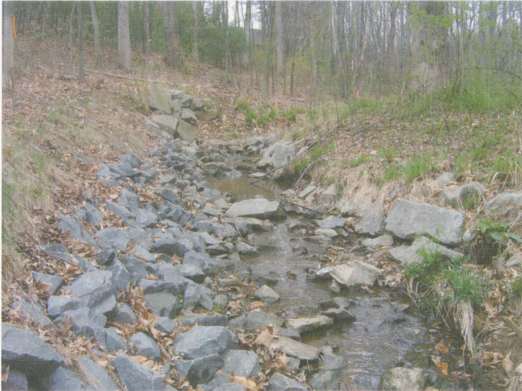
5. Looking northwest (upstream) at Reach 1-E of Snakeden Branch on the western portion of the study area.
