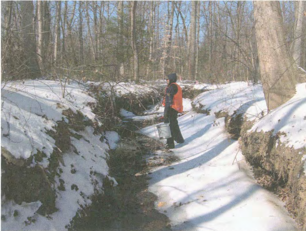
3. Looking west (upstream) at Reach 3-A of Colvin Run in the southern portion of the study area.
