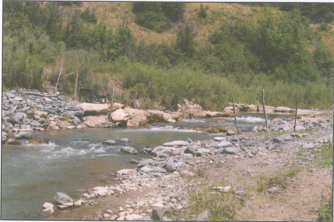
PHOTO 1. LOOKING UPSTREAM AT A 3 - STEP CROSS VANE .
