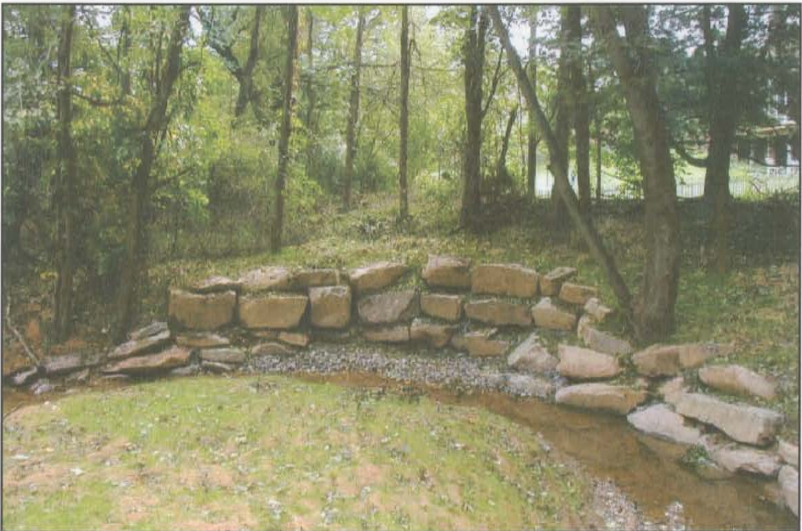
PHOTO 2. IMBRICATED RIPRAP ALONG THE MEANDER OF A PERENNIAL STREAM IN NORTHERN VIRGINIA.
