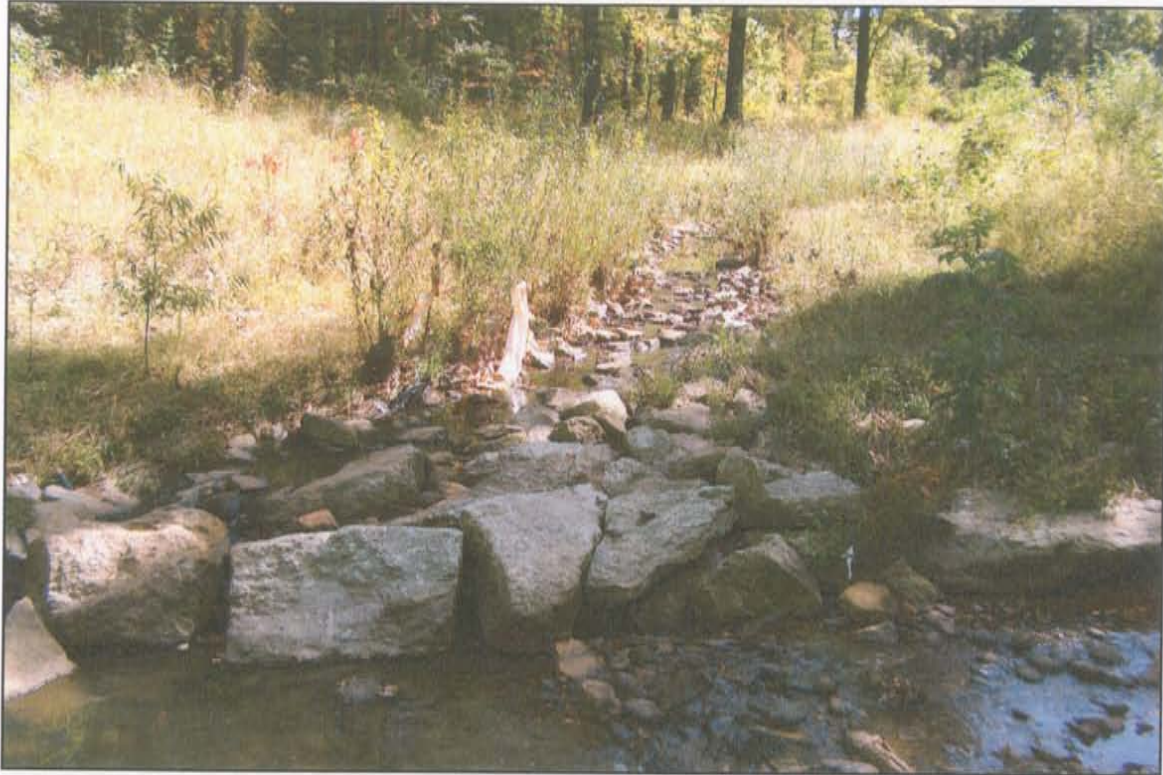
PHOTO 1. REINFORCED STREAM BED WITH STABILIZATION AT CONFLUENCE.
