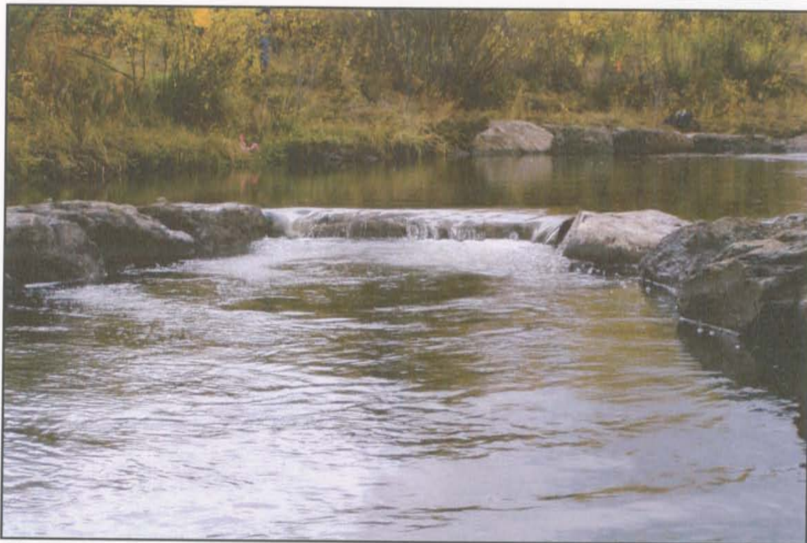
PHOTO 1. LOOKING UPSTREAM AT THE WEIR SECTION OF A CROSS VANE AT LOW FLOW.
