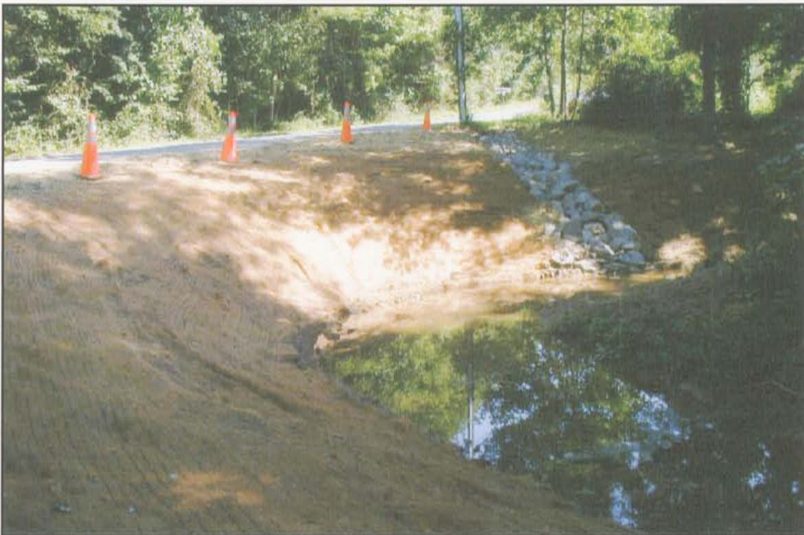
PHOTO 2. A RECENTLY CONSTRUCTED STREAM RESTORATION PROJECT UTILIZING COIR LOGS WITH MATTING.
