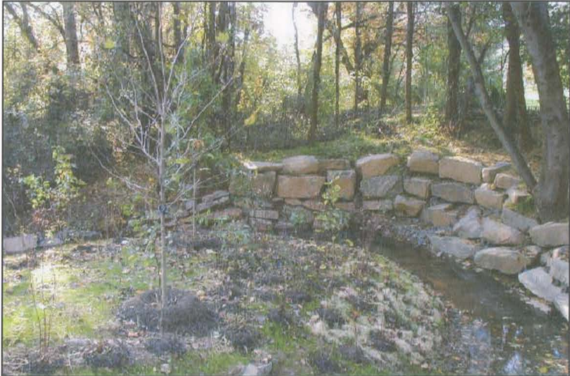
PHOTO 1. IMBRICATED RIPRAP ALONG THE MEANDER OF A PERENNIAL STREAM IN NORTHERN VIRGINIA.
