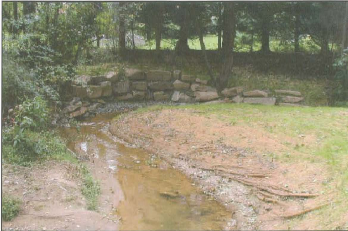
PHOTO 1. COIR LOGS WITH MATTING PLACED ALONG THE RIGHT BANK OF THIS NORTHERN VIRGINIA STREAM.
