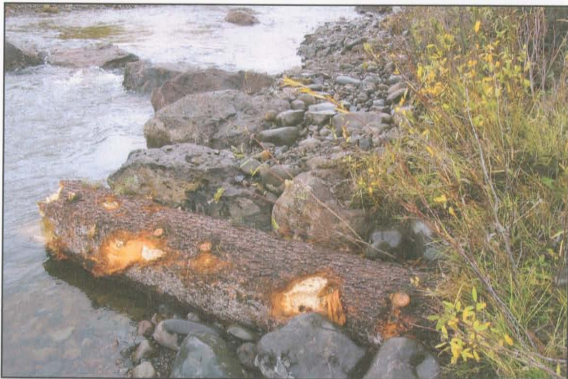
PHOTO 2. J-HOOK WITH A ROCK AND LOG SILL ON THE EXTENDING FROM THE "HOOK."
