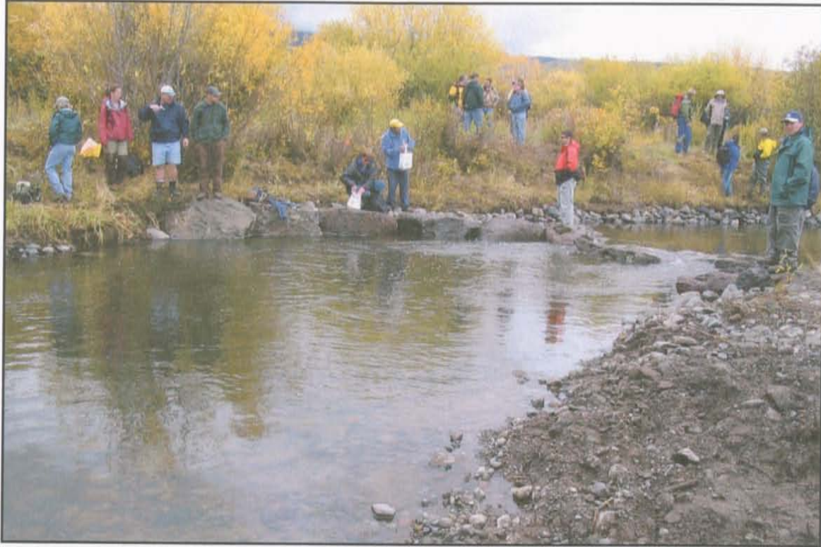
PHOTO 1. A J-HOOK WITH SILL PLACED IN A MEANDER TO PROTECT THE OUTER STREAMBANK AND TO HELP MAINTAIN THE STREAM'S RIFFLE/POOL SEQUENCE.
