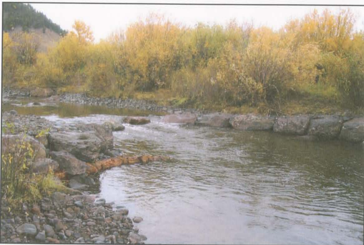
PHOTO 2. LOOKING UPSTREAM AT WATER FLOWING OVER THE WEIR SECTION OF A CROSS VANE AT LOW FLOW. VANE ARMS ARE SHOWN EXTENDING TO BANKFULL.
