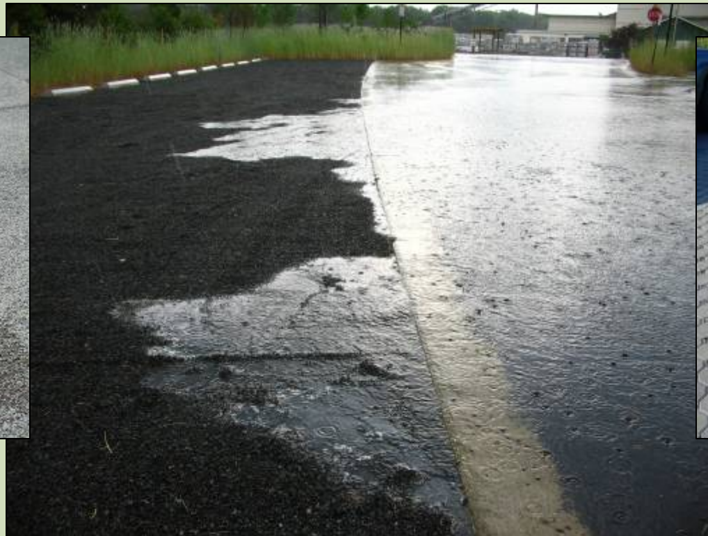
GravelPave2 infiltrating during a large rain storm at WSSI
