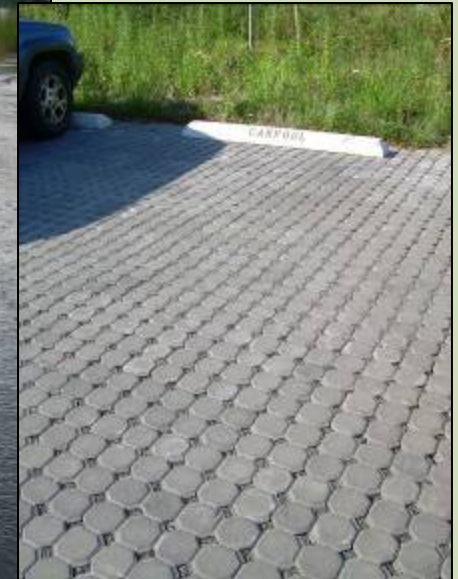
Pervious pavers at WSSI
