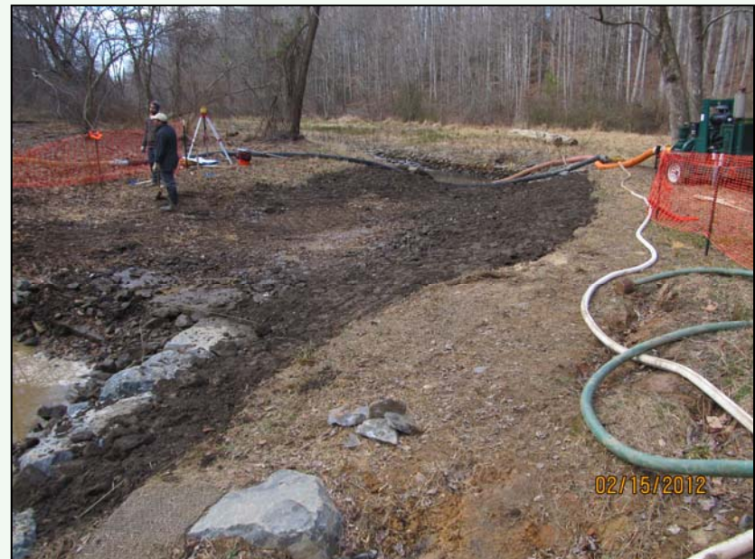
Rock wall and channel grading commenced
