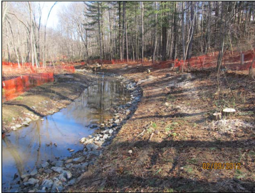
Tree clearing complete
