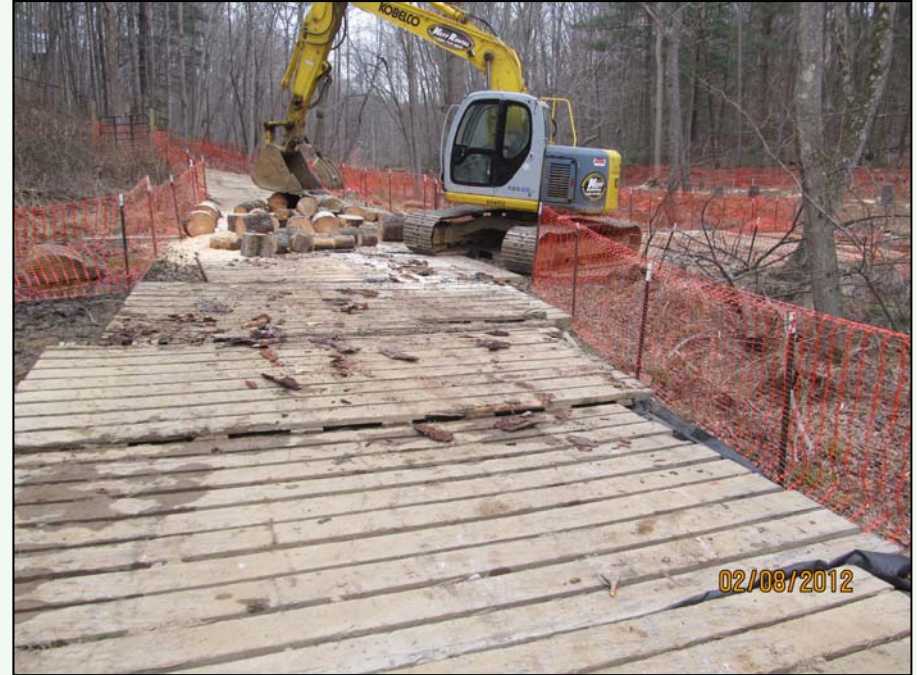
Deck Mats used in active cut-ins
