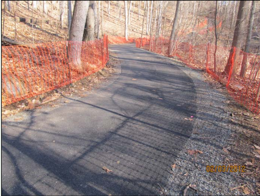
Tree protection fencing installed, early February
