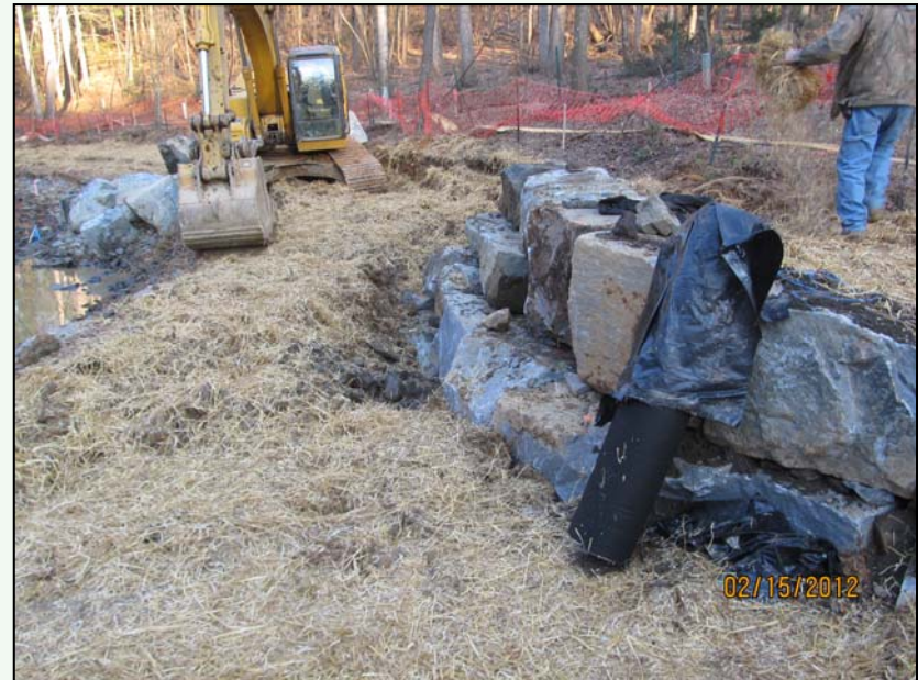
Rock wall and channel grading commenced
