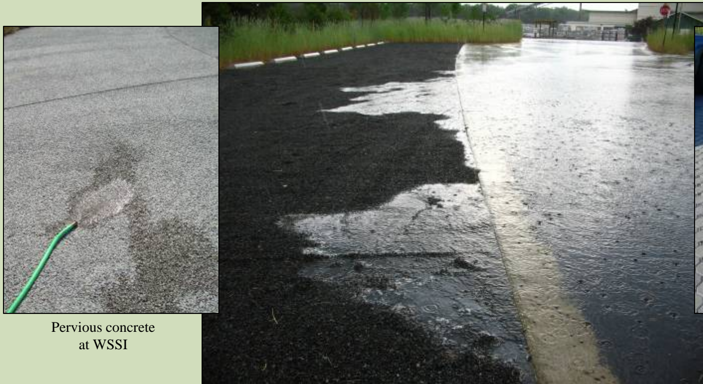
GravelPave2 infiltrating during a large rain storm at WSSI
