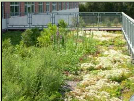
Green roof at WSSI
