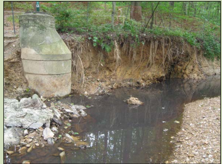
Exposed sewer manhole – Reach 12 in Snakeden
