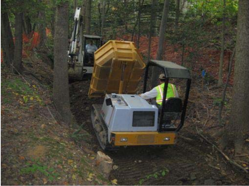
Figure 5. Reach 8A – Construction with minimal disturbance
