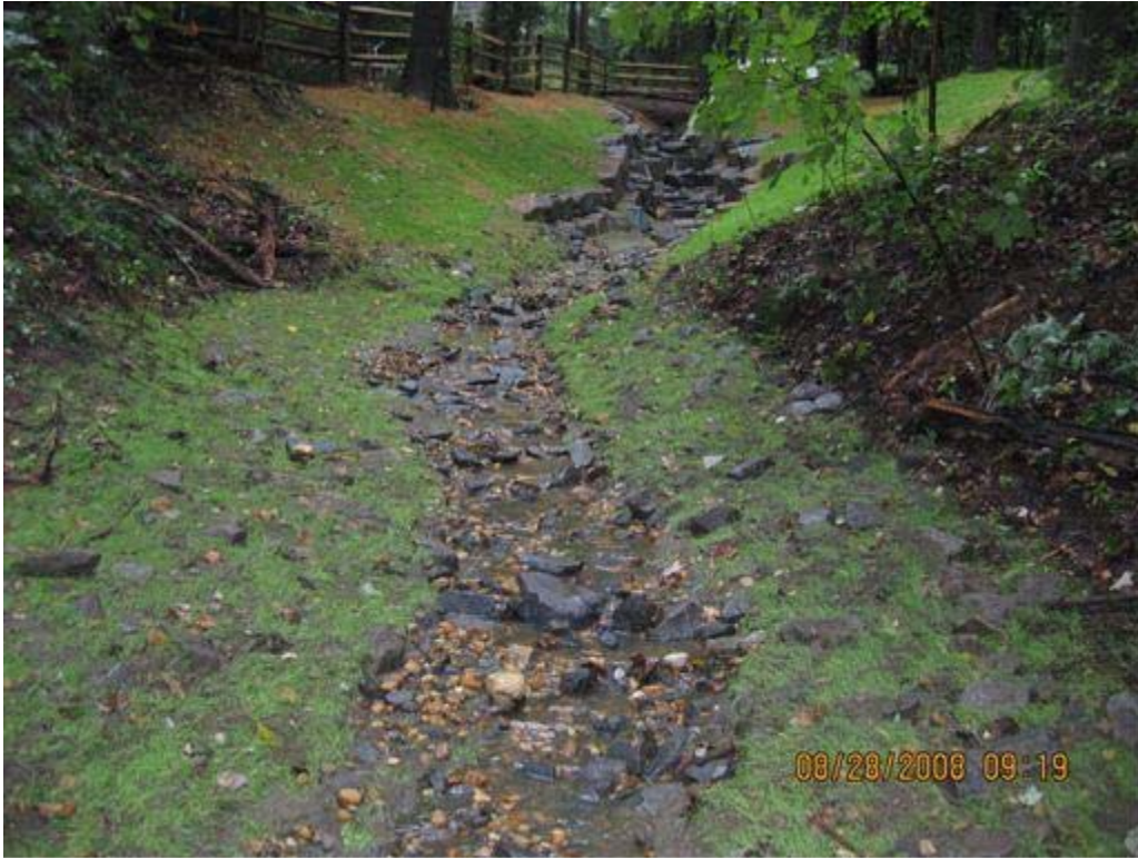
Figure 7. Reach 10 –after construction
