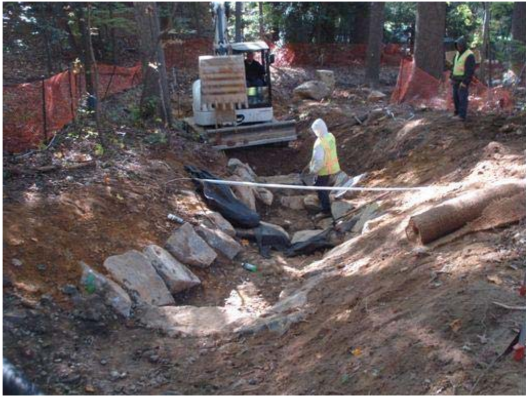
Figure 4. Reach 8 – During Construction
